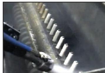
Soda blasting is ideal for cleaning all types of delicate equipment and surfaces.
