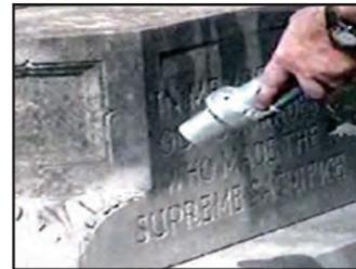
From painted concrete to soft limestone monuments, soda blasting knows no equal. Because of the non-destructive abrasive effect of soda blasting, either hard or soft masonry and stone surfaces can easily be cleaned in a matter of minutes.
