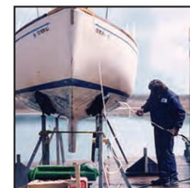
When bottom paint has areas where the anti-fouling paint has thinned or exhibits oxidation, but the overall paint condition is good, a "sweep blast" can be performed to remove surface contaminants and rejuvenate the paint for touch up painting or vessel launching.
